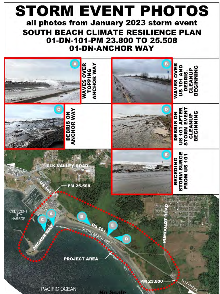
Figure 1: Project Area and Storm Damage photos
