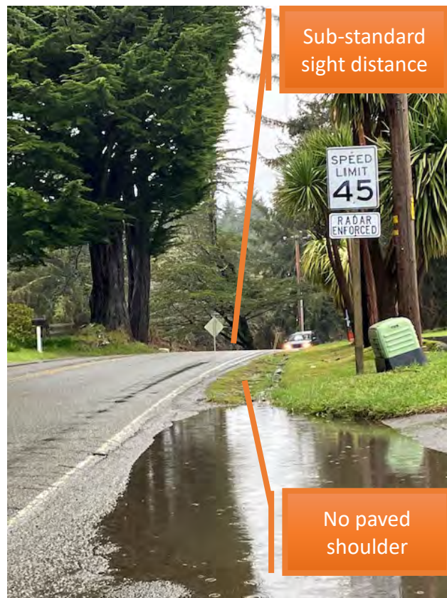
Figure 1: Elk Valley Road at Howland Hill Road intersection, looking north
