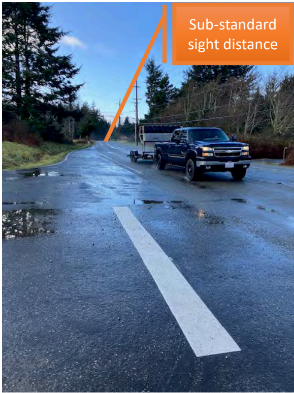
Figure 6: Elk Valley Road at Aubell Lane, looking south
