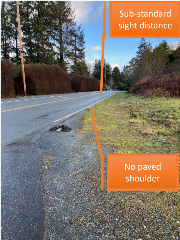
Figure 7: Elk Valley Road at Aubell Lane, looking north
